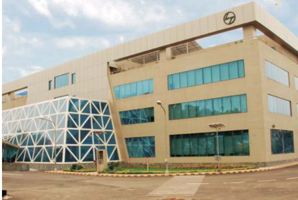
Switchgear Factory, Navi Mumbai
