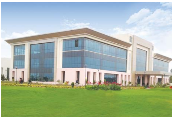
Switchgear Factory, Vadodara
