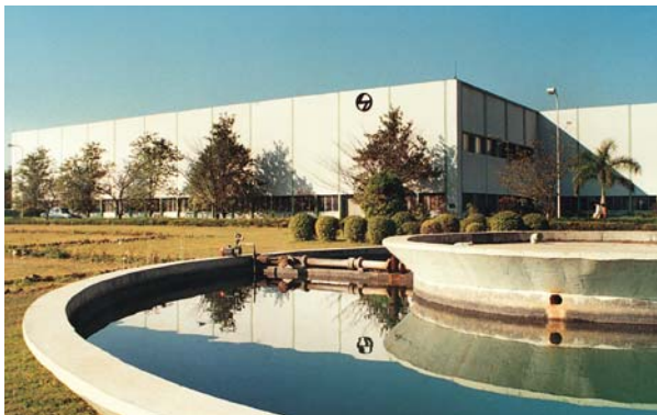
Switchgear Factory, Ahmednagar
